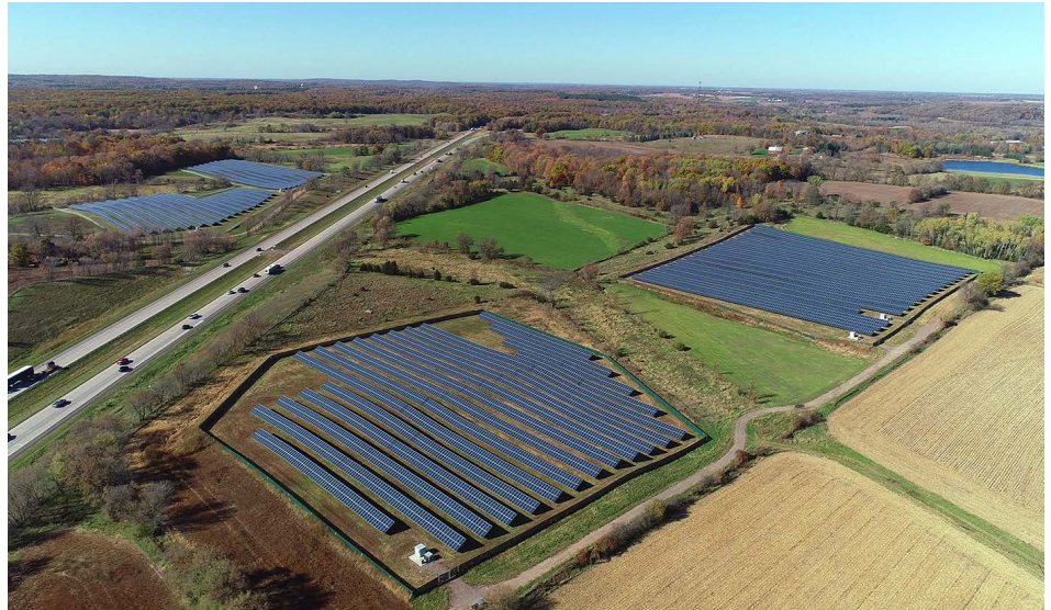
ST. JOSEPH COMMUNITY SOLAR GARDEN, MN | CREDIT: IMPACT POWER SOLUTIONS
