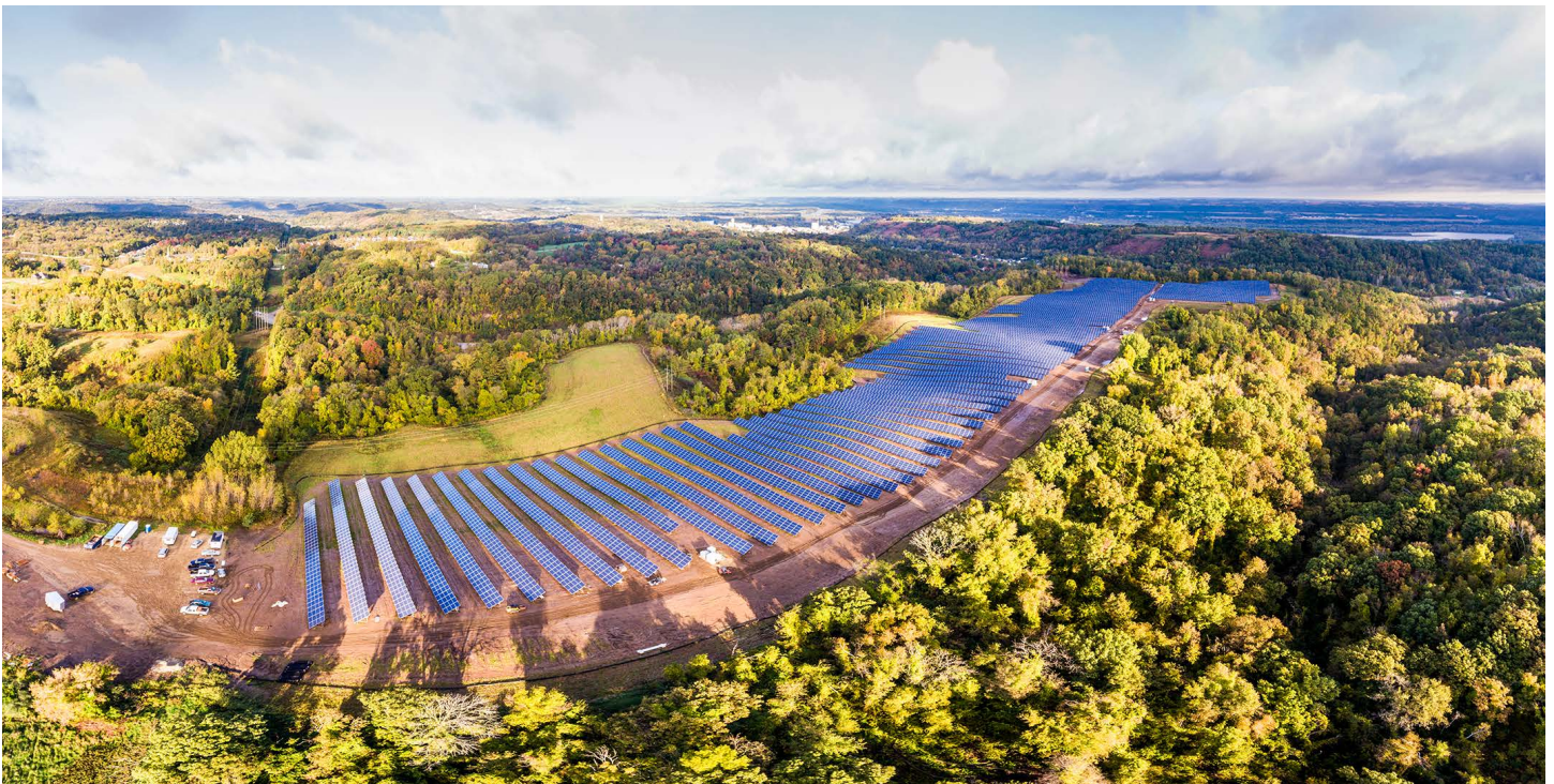
RED WING COMMUNITY SOLAR GARDEN, MN | CREDIT: IPS SOLAR
